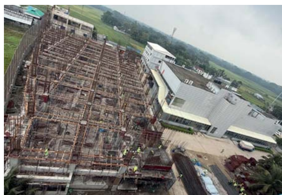
Under Construction of the New Generic Building
